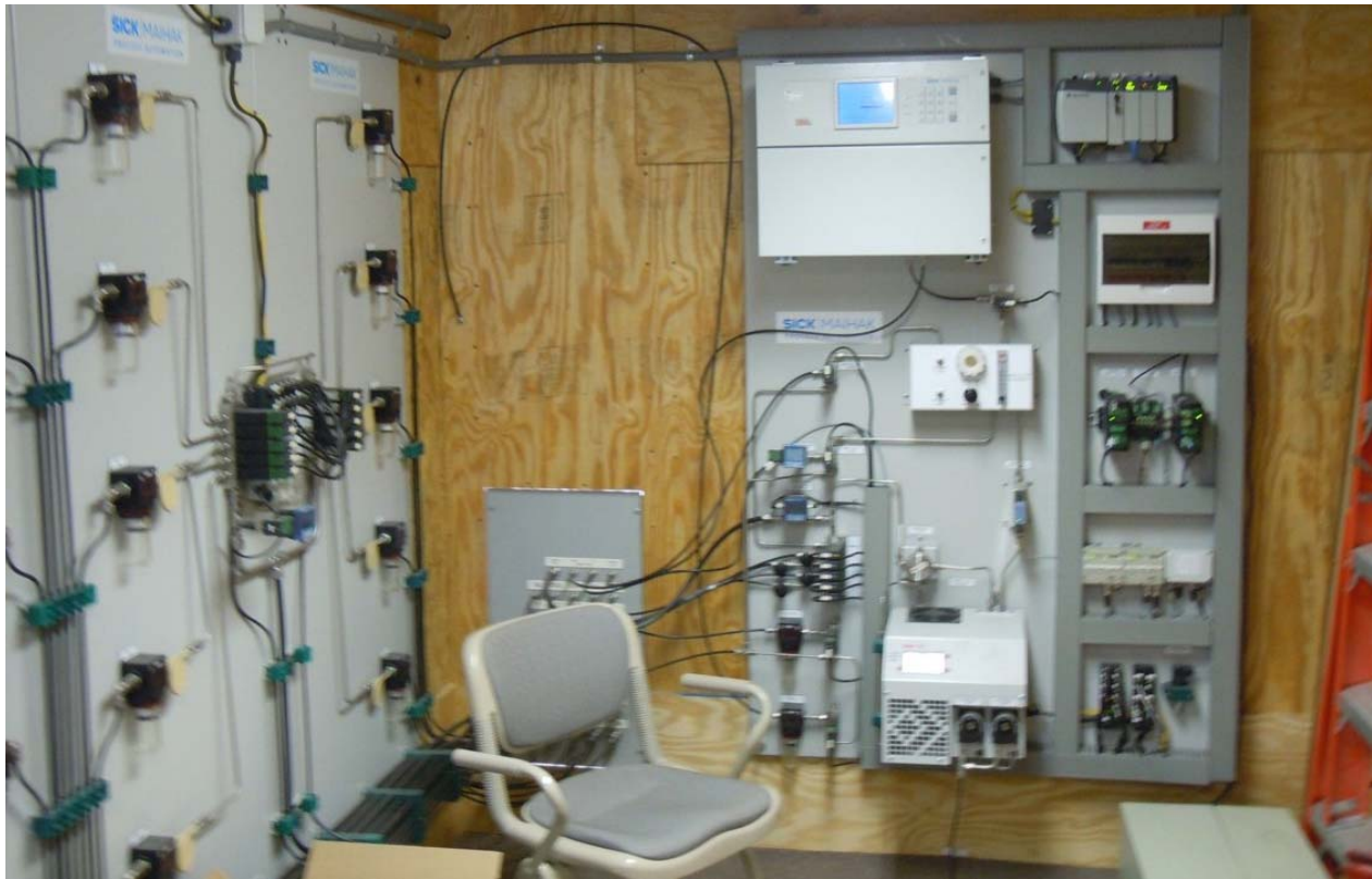
Figure 3.3. Inside of a sampling trailer with analyzer shown in top middle.
