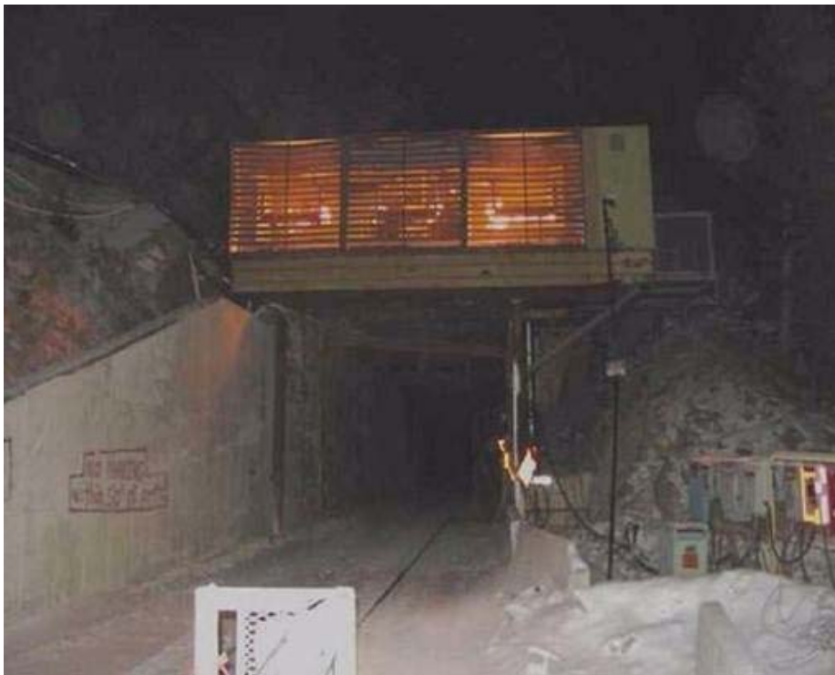
Figure 6.1: Typical direct-fired air heater mounted over the intake portal.
