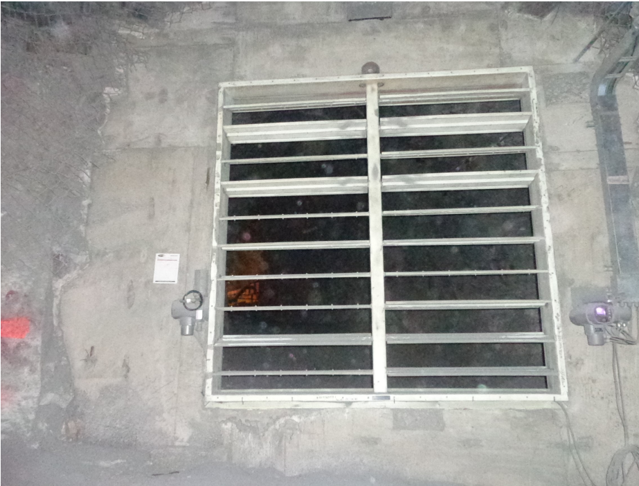
Figure 4.11: Louver regulator in an underground Copper Mine.
