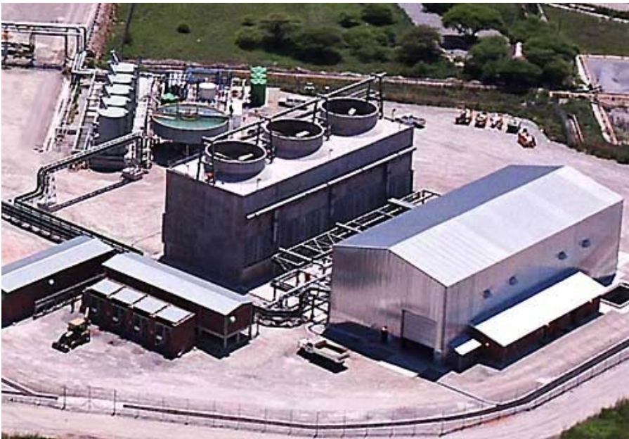
Figure 4.1: Modern, mine refrigeration plant including cooling towers. (Mining Technology).
