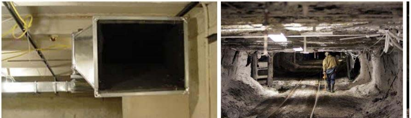
Figure 4.1. Typical mine openings (right), compared with a more uniform HVAC duct. It is evident that the mine openings have relatively high frictional losses.
