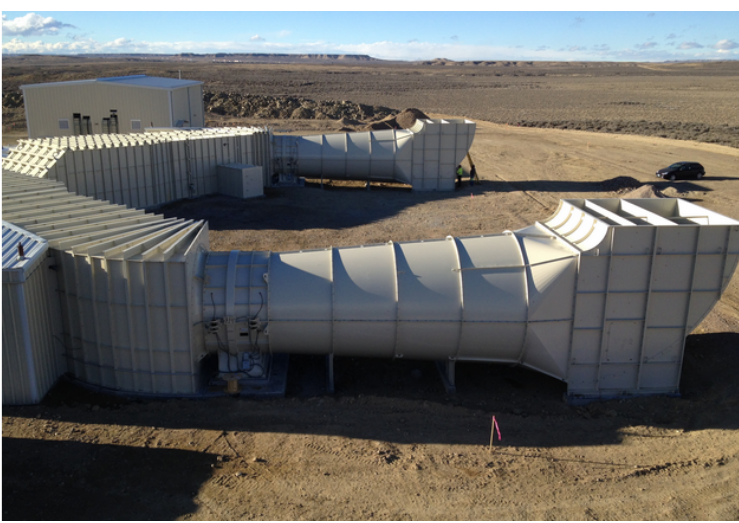
Figure 2.3. Major external components of a fan housing, including the evase and directional ducting
