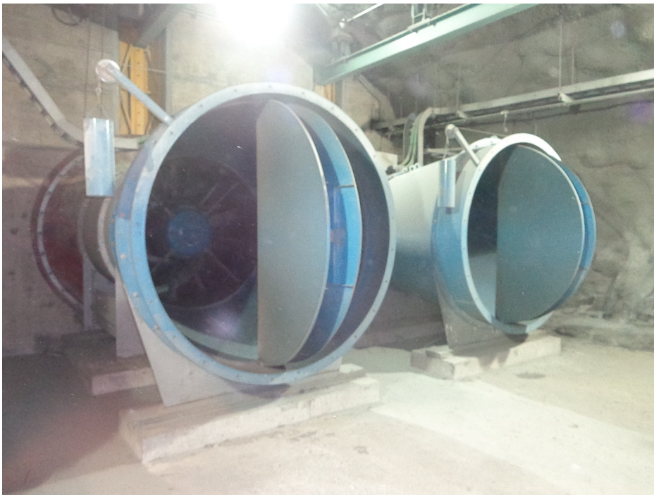
Figure 4.17: Underground booster fan installation showing backflow dampers (outlet side).
