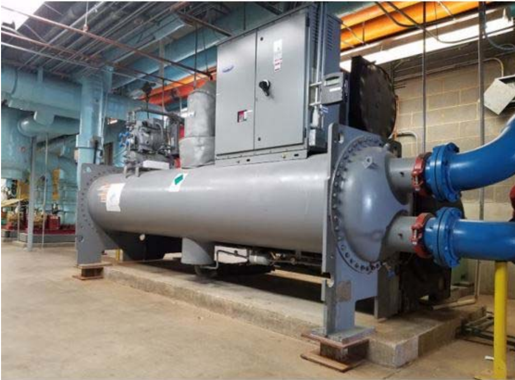
Figure 4.3: 400-ton Chiller (Carrier).
