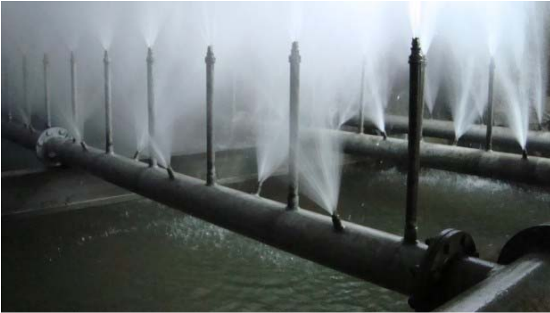
Figure 5.3: Inside view of a spray chamber (BBE).
