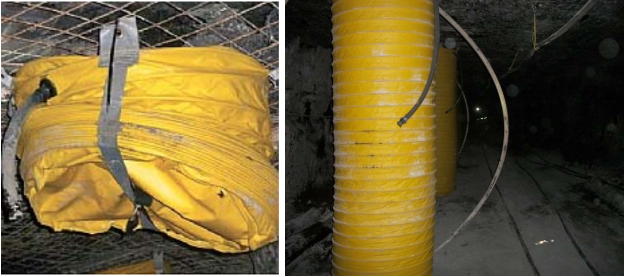
Fig. 1: (a) Crib bag installed in a collapsed configuration to the mine roof; and (b) Crab bag after filling with cementitious material (from Jennmar 2013; NTI 2019)
