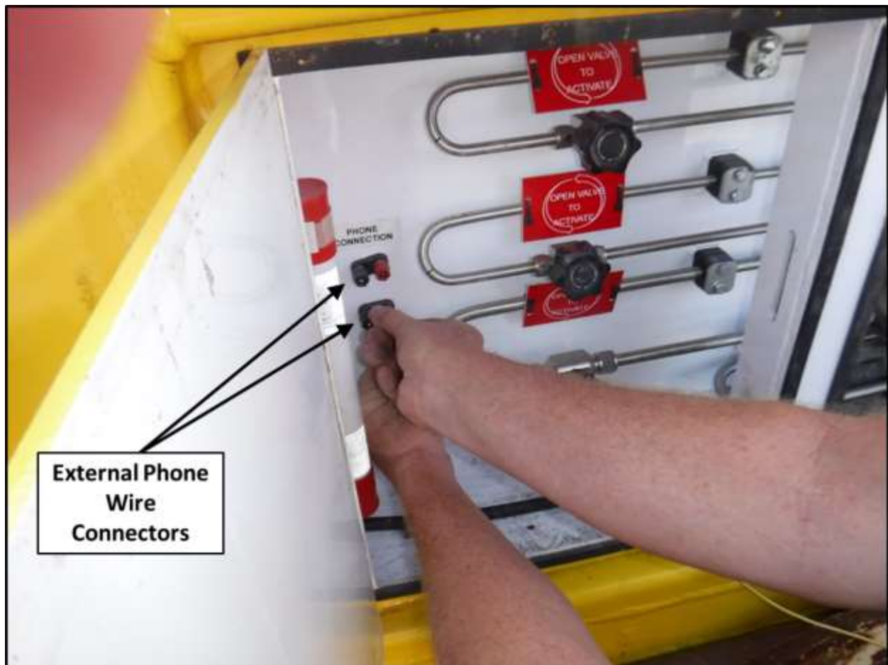
Figure 30: Location of external connectors for standard hard-wired mine pager phones.
