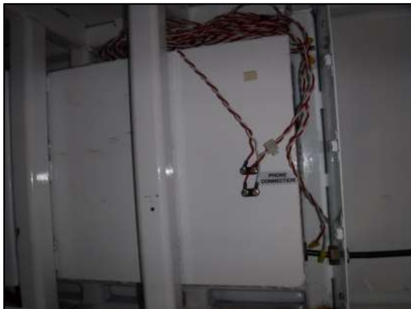
Figure 31: Standard pager phone connectors inside the inflated refuge compartment.
