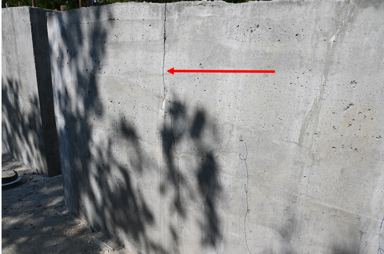
Figure 4.4. Crack on Rear Surface Extending Down from the Top
