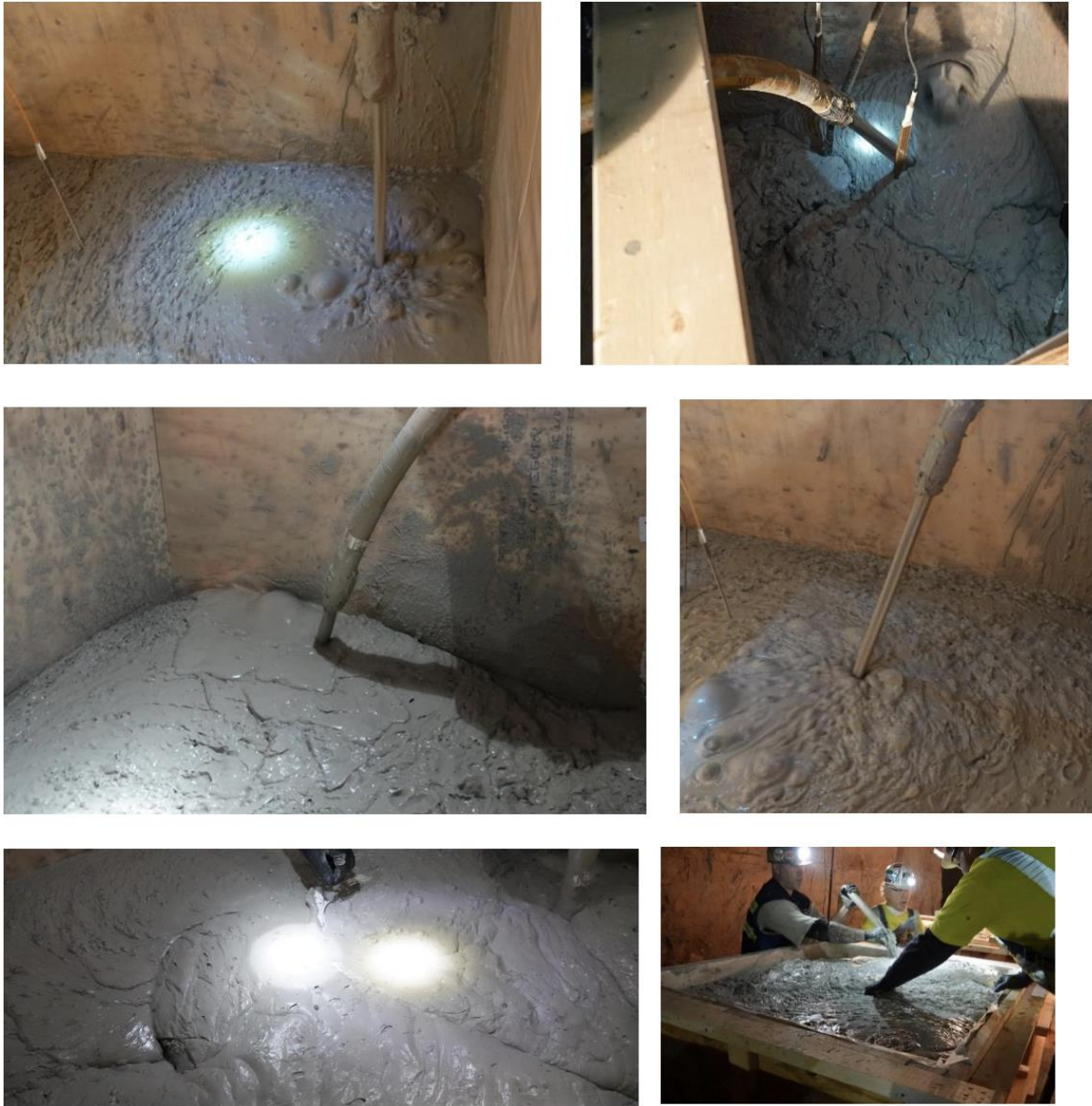
Figure 3.18 Pouring of Mixtures A and B into the wooden forms
