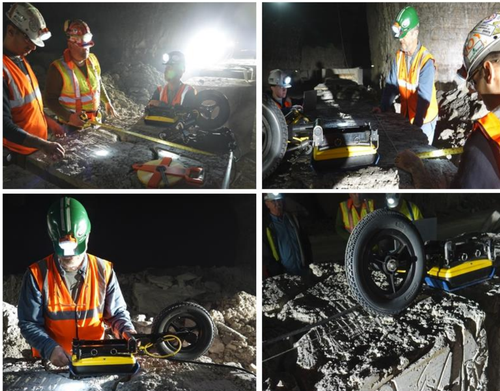
Figure 3.26 Collection of the GPR information
