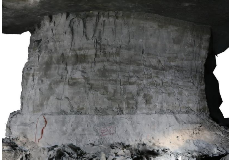
Figure 44 Initial pillar photogrammetry model at east Tennessee mine
