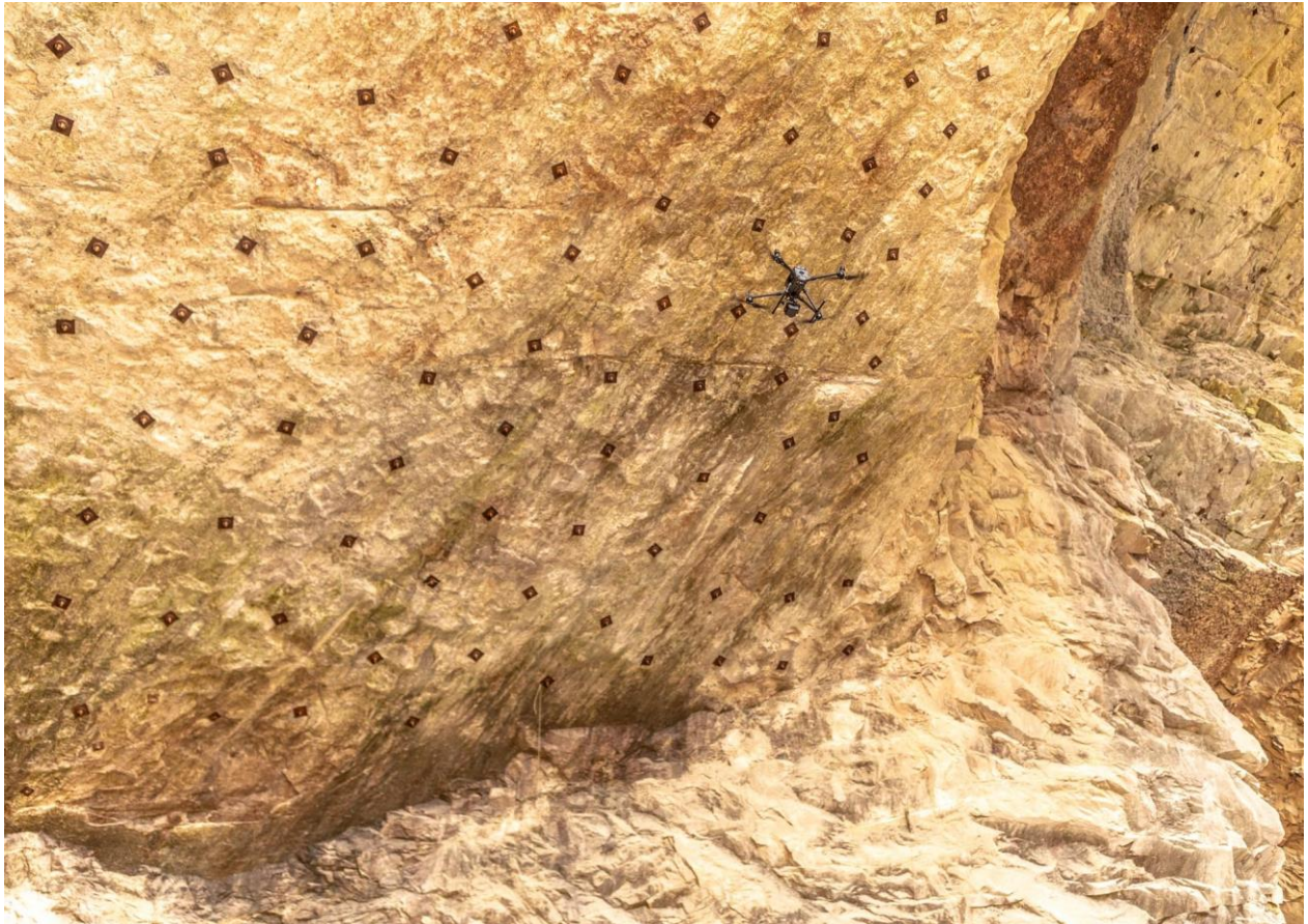
Figure 34 Drone-based roof & roof bolt inspection
