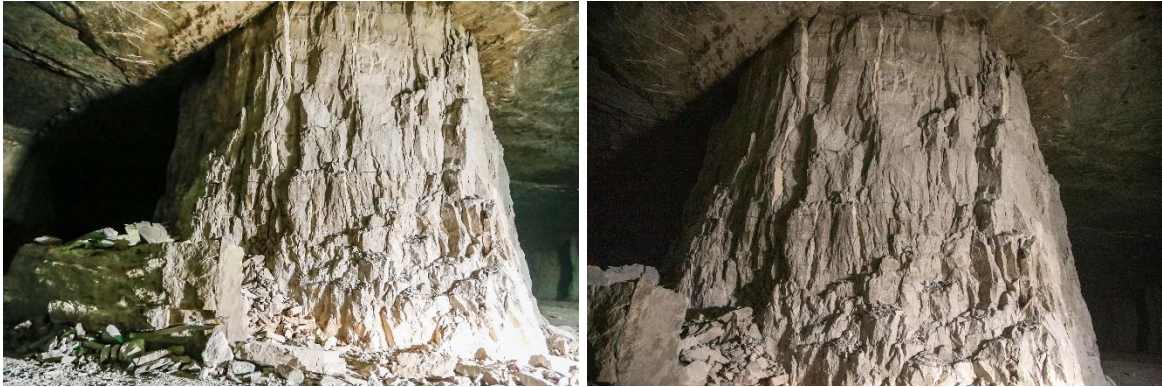
Figure 42 Example mine pillars at a limestone mine in east Tennessee
