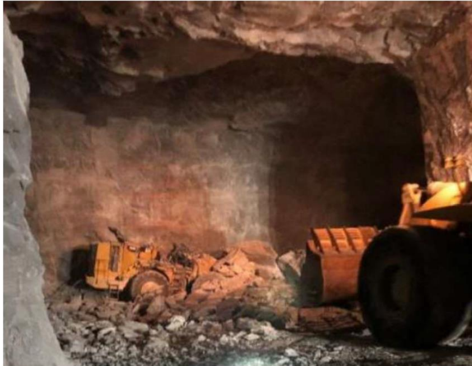
Figure 3 Roof fall fatality in PA (MSHA, 2022b)
